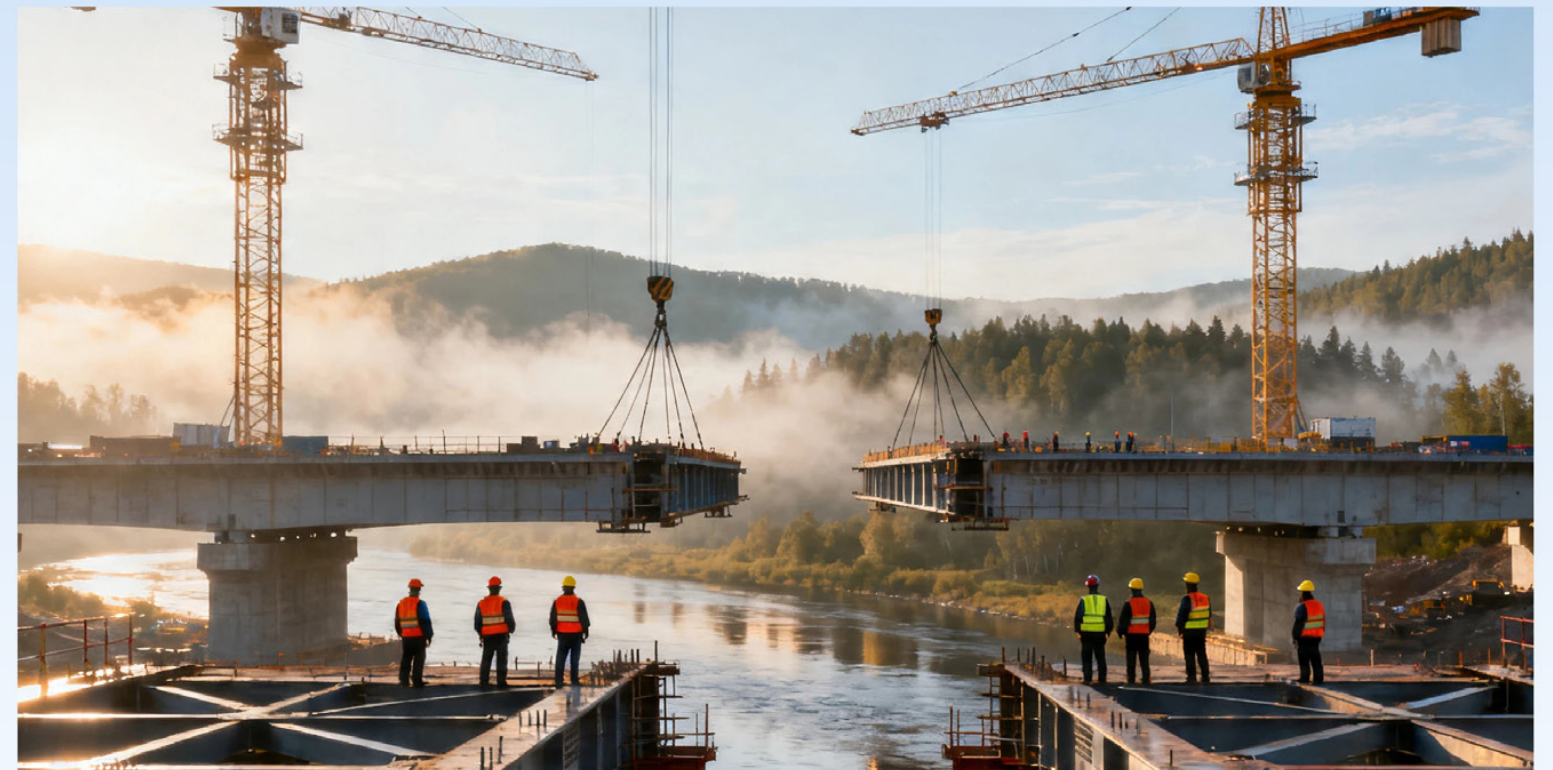
Both sections of the DPRK-Russia border motor bridge connected
